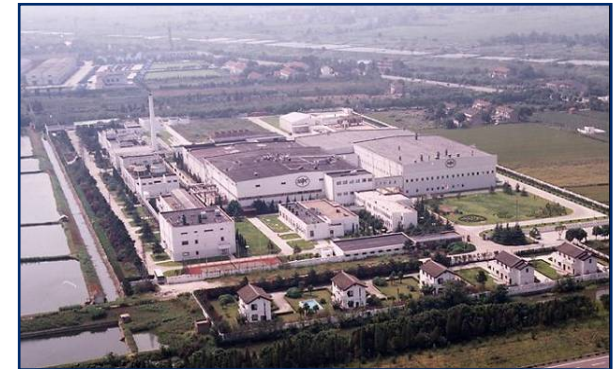
Wuxi: Clinical Nutrition, R&D site (under construction)
